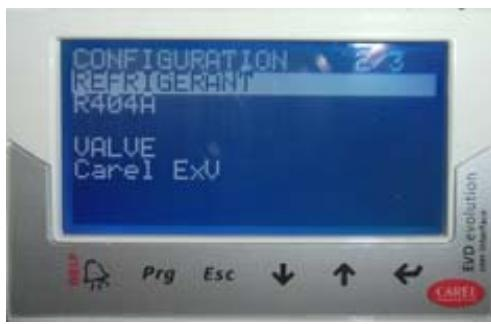
4. Select **REFRIGERANT** and push the Enter Button ↴ then the "Arrows up-down" till the **Refrigerant R744**.
